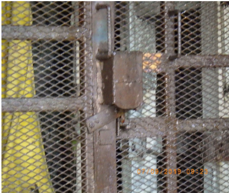
Left - The latch to the main portal is open has been left unsecured/locked. Right – The main portal.
